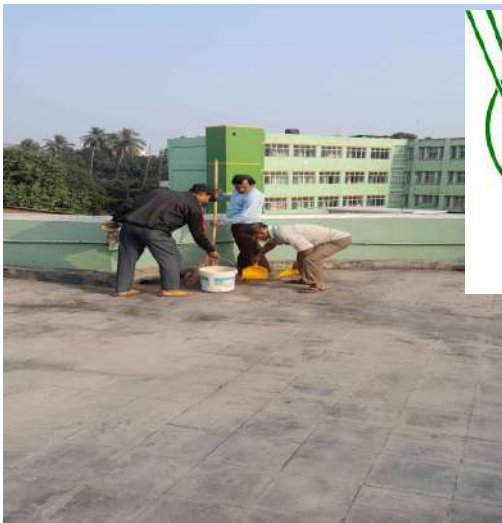
Cleaning of Roof top
